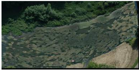
Fig. 41 : Our test site (Izel) from the sky. Picture taken on june 2008. The white spot is the calibration system (Fig. 40)
